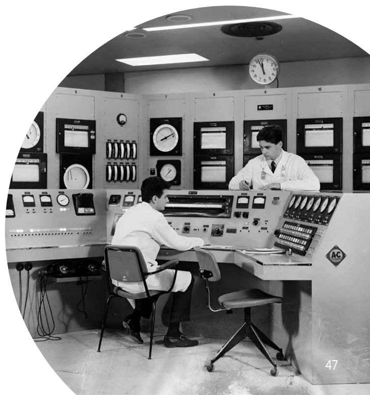
Nuclear research facilities in Ispra, 1960 (Italy)
