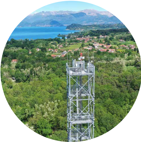
Atmospheric Observatory Tower JRC Ispra site (Italy)
